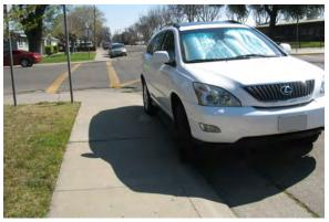
A car parked on the sidewalk due to a rolled-edge curb.
