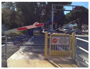
Detecable warning surfaces and pedestrian gates placed on sidewalk approaching railroad tracks
