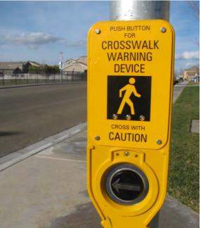
**Top and Above** An in-pavement lighted crosswalk and a push button to activate the warning sign.
