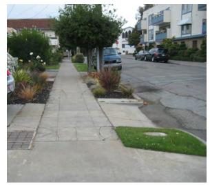
*Optimal driveway design provides a smooth and continuous sidewalk with the driveway apron at the street edge within the planting strip*
